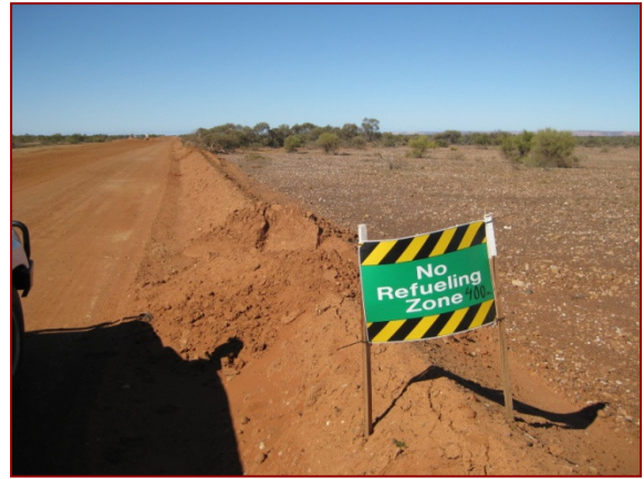
No refuelling signage adjacent to watercourse crossing
