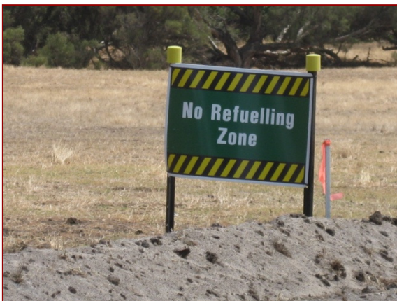
No refuelling signage adjacent to wetland crossing
