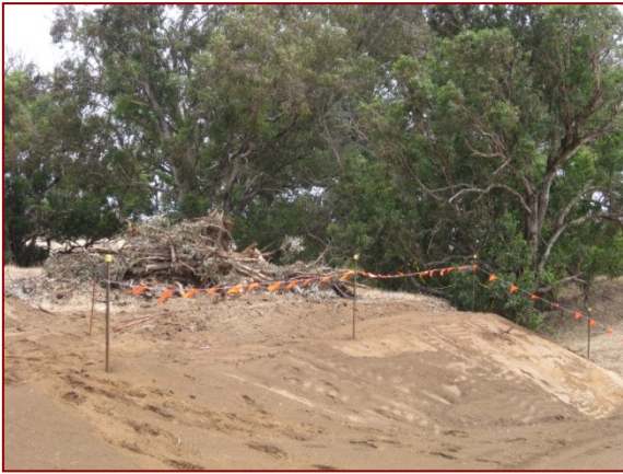
Riparian vegetation stockpiling and delineation of area
