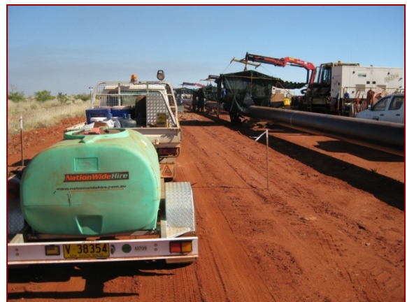
Fast attack fire control trailer available with welding activities
