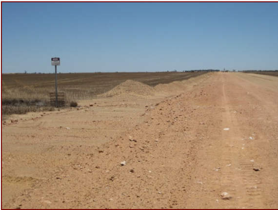
Topsoil stockpile retained after backfilling, prior to respreading
