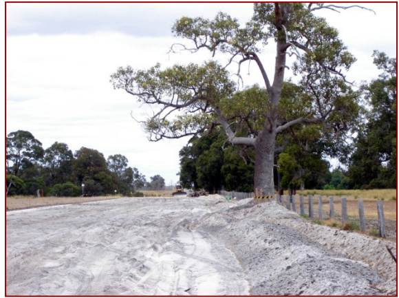
Retained tree overhanging CROW
