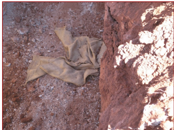
Hessian fauna refuge at base of trench
