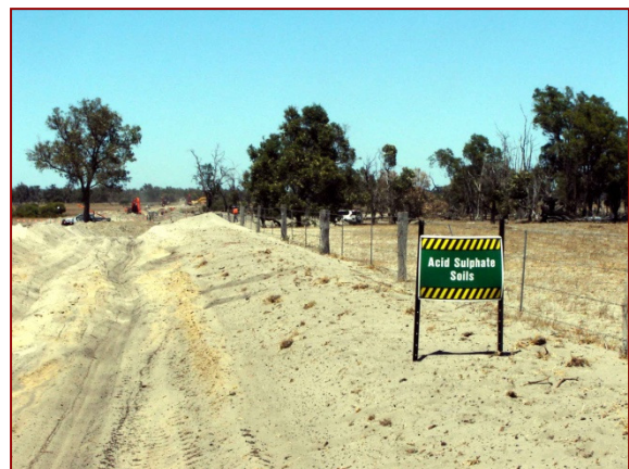
Acid sulphate soils area demarcation signage
