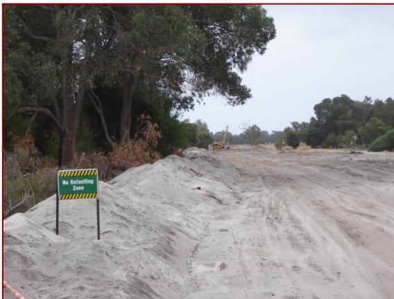
No refuelling signage adjacent to wetland crossing
