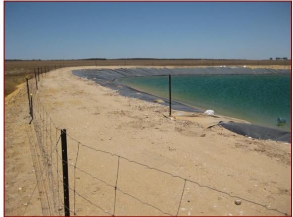
Turkey nest dam located in cleared farmland
