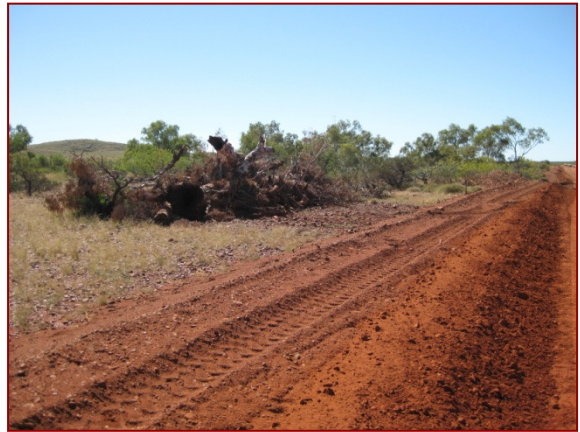
Vegetation stockpile adjacent to CROW source area
