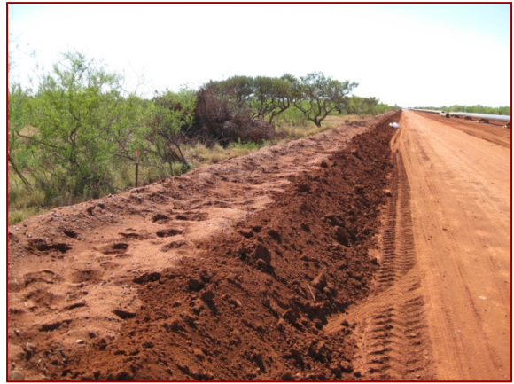
Topsoil stockpile adjacent to CROW source area
