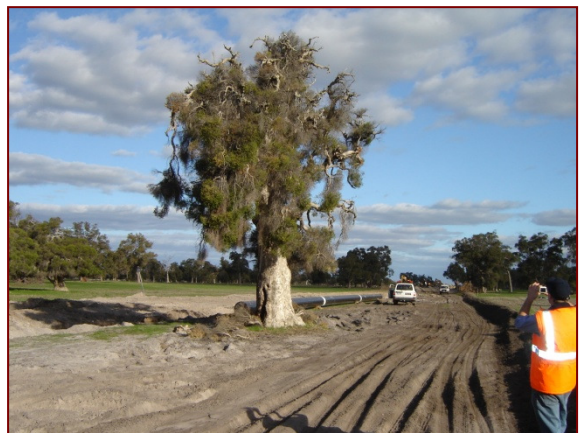
Retained habitat tree on edge of CROW
