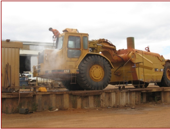
Plant washdown prior to transfer to site
