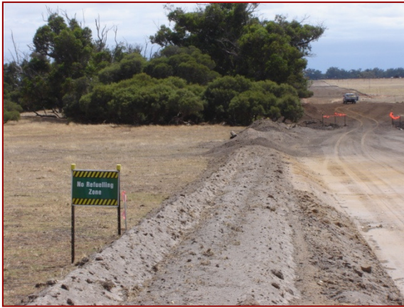
No refuelling signage adjacent to watercourse crossing
