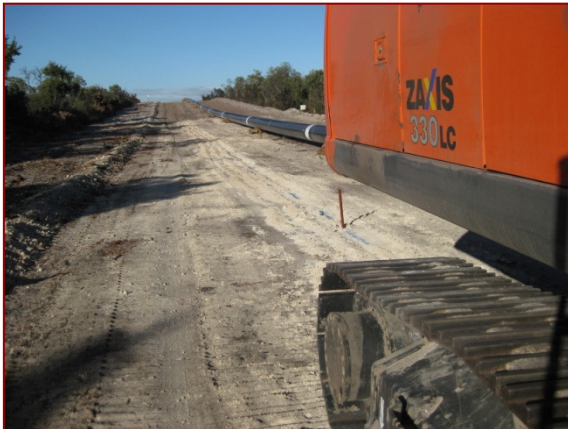
Neutralising agent (aglime) laid on pipeline alignment prior to trench excavation
