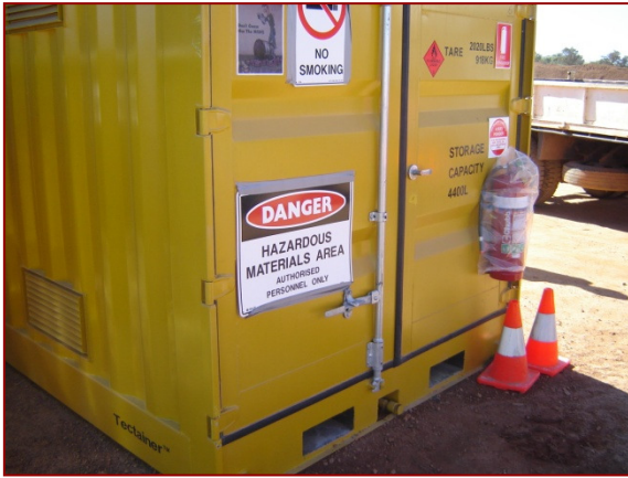
Hazardous material storage container and signage
