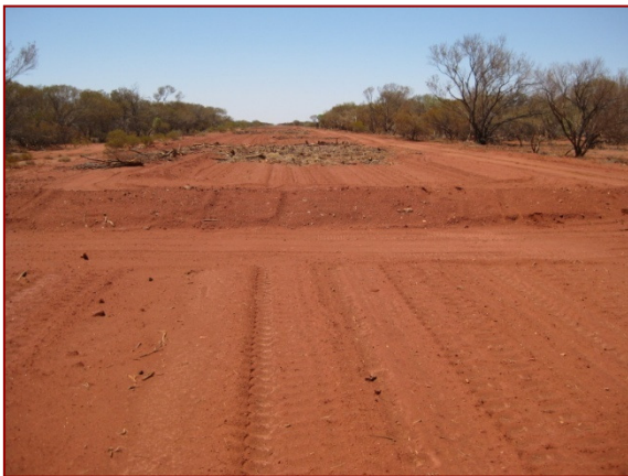
Erosion protection berm across rehabilitated CROW
