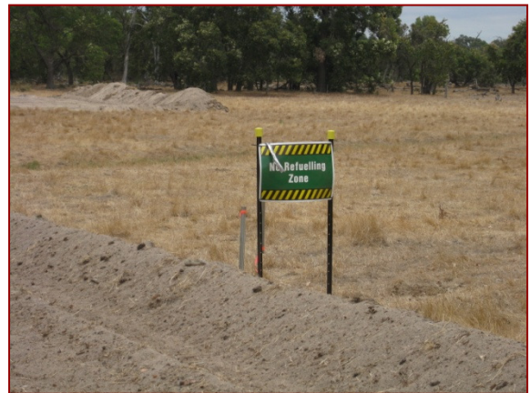
No refuelling signage adjacent to wetland crossing
