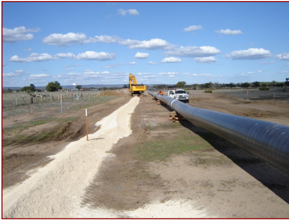
Neutralising agent (aglime) laid on pipeline alignment prior to trench excavation
