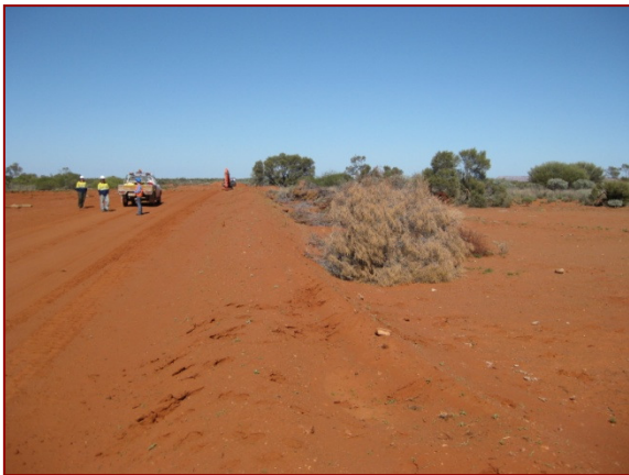
Vegetation stockpile adjacent to CROW source area, separate from topsoil stockpile
