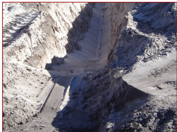
Fauna exit ramp and trench plug
