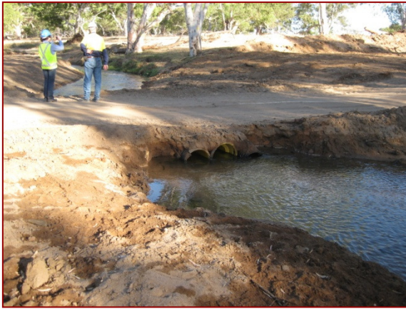
Watercourse crossing flumes to maintain downstream flow regime
