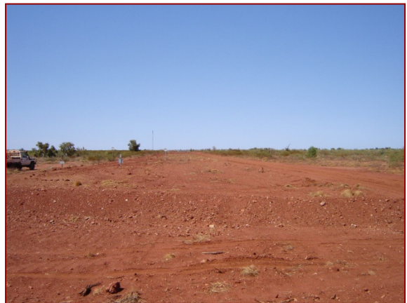
Erosion protection berm across rehabilitated CROW
