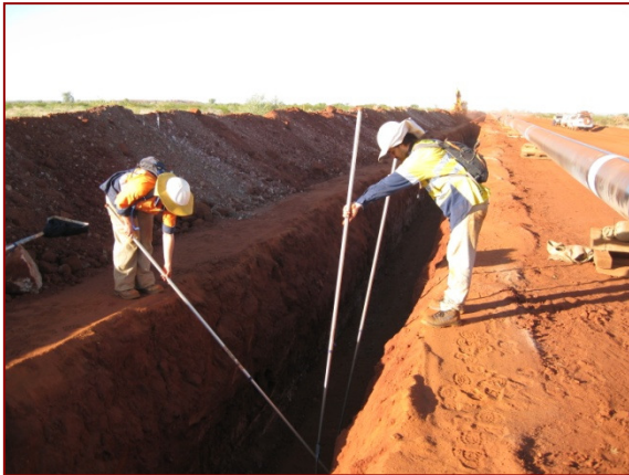
Fauna clearing team removing entrapped fauna from trench
