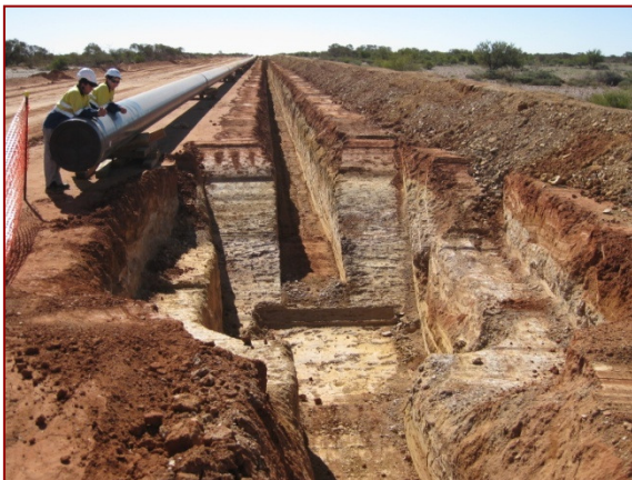
Fauna exit ramps at 45° slope to trench plug
