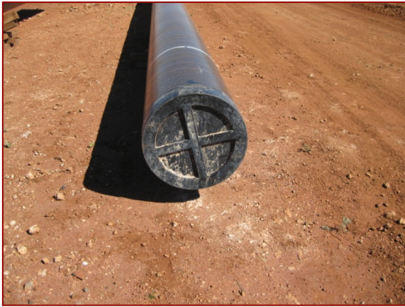
End caps on welded pipe to prevent fauna entry and entrapment
