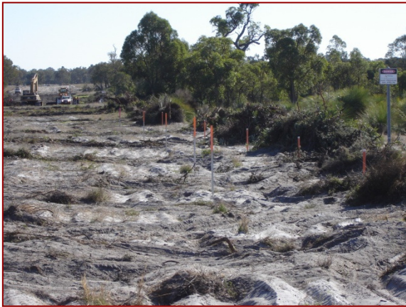
Vegetation stockpile adjacent to CROW source area
