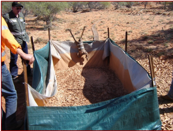
Dewatering discharge sediment trap
