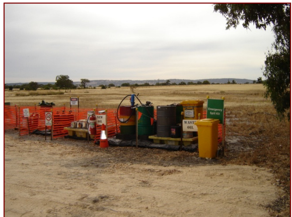
Material storage area in construction yard in cleared farmland
