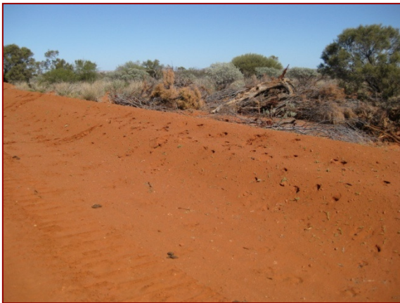
Topsoil stockpile adjacent to CROW source area, separate from vegetation stockpile
