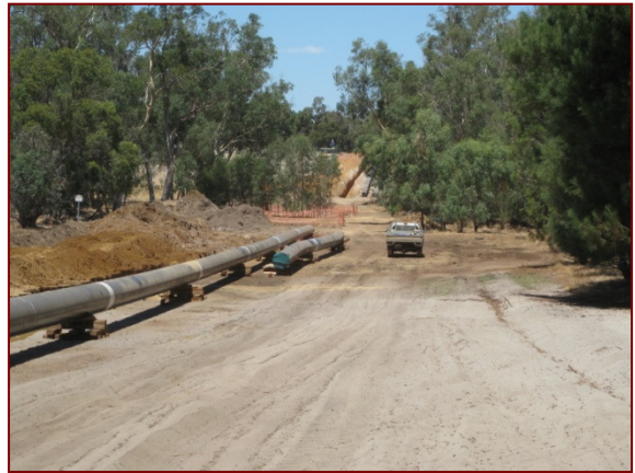
Horizontal drilling location at Caren Caren Brook looking across watercourse
