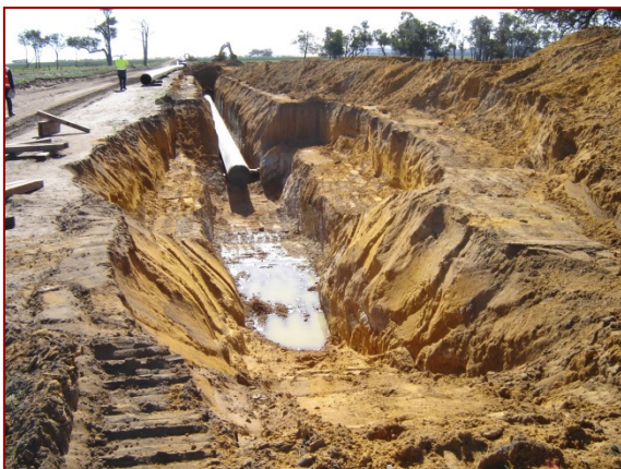
Fauna exit ramp and trench plug
